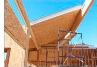
Structural insulated panel
